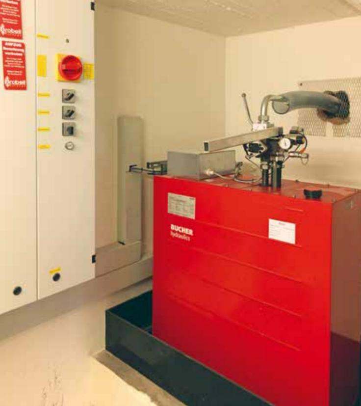
Detail: Hydraulik Aggregat
